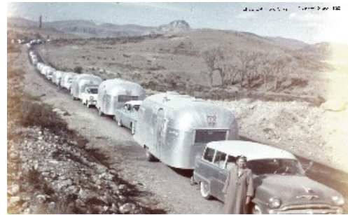
1957 Mexican Caravan - gas line
