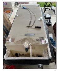
Looking from underneath, the repaired pex piping and low point drains moved inside ready for the tank and insulating shell to be installed
