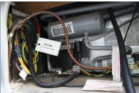
5: Lower Refrigerator Access Opening (Note Wiring Tag Labeled 24 Volts)
