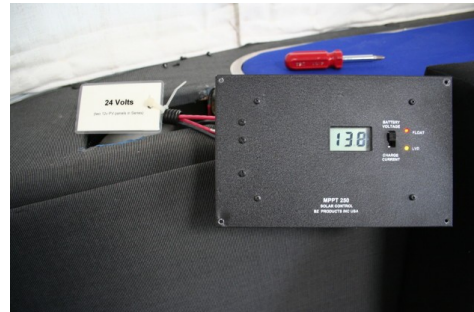
6: System Installed and Float Voltage Set (Note Wiring Tag Labeled 24 Volts)
